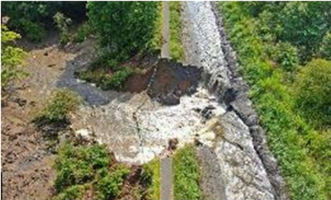
Union Canal east of Linlithgow – breach 2020, repair, adaptation
