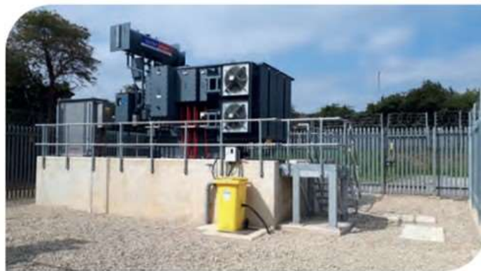
Elevated substation at Drakes Way
